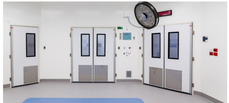
Altro Whiterock in an operating room
