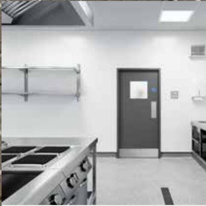
Fire performance: hygienic wall coverings to Class B-s3 d0, hygienic doorsets to FD60
