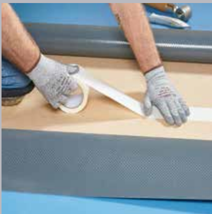
Tape perimeter and seams
